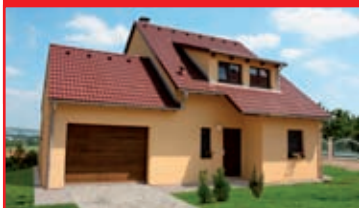
Novostavba RD Provodov u ZL
