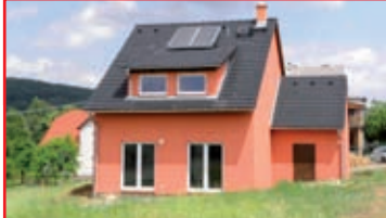
Novostavba RD Provodov u ZL
