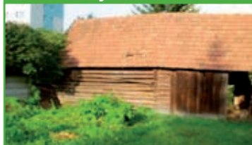
Brumov - Bylnice N05240
